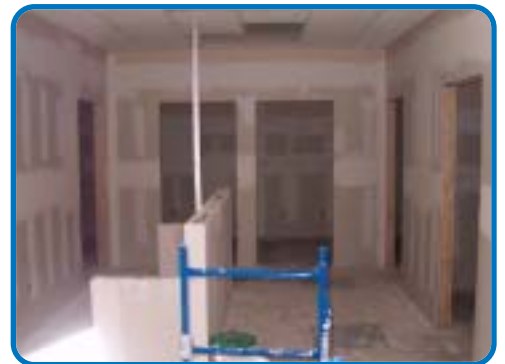
With new sheetrock, the clinic begins to take shape.
