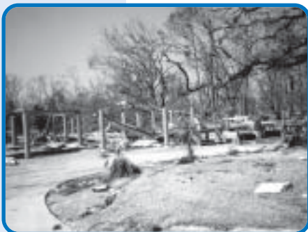
The hurricane ripped this building off its foundation.
